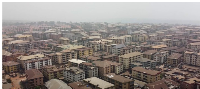
Figure 1: High housing density in close proximity to each other at Onitsha in Anambra State, Nigeria.
